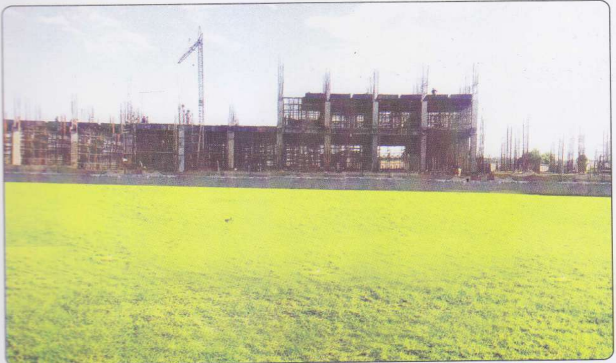
Work in progress at New PCA Stadium Mullanpur, New Chandigarh
